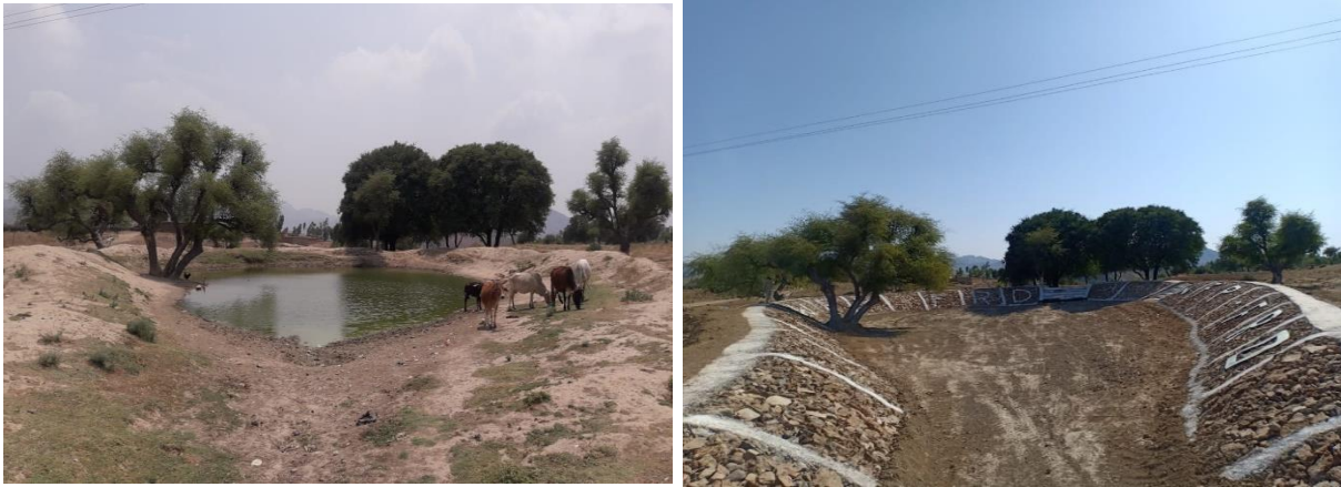
Figure 27. Stone Pitching/improvement of water reservoir with a height of less than 3m and a storage capacity of less than 400m 3 .
