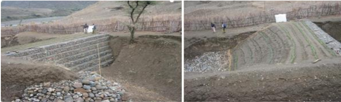
Figure 26. The rehabilitation and transformation of a gully land into productive units by building soil sedimentation and overflow structure, gabions and weirs are possible across large gullies- having less than 3m high/depth OR have a storage capacity of less than 400m 3
