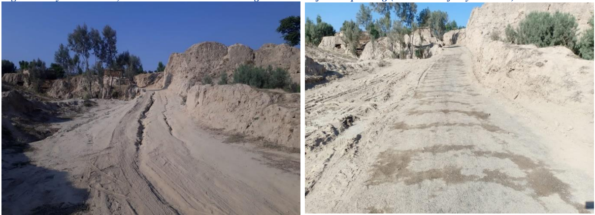
Figure 29. Improvement of Physical access/gully control by stone pitching/other ingenious techniques without cutting and altering the natural land as well as land cover of forests
