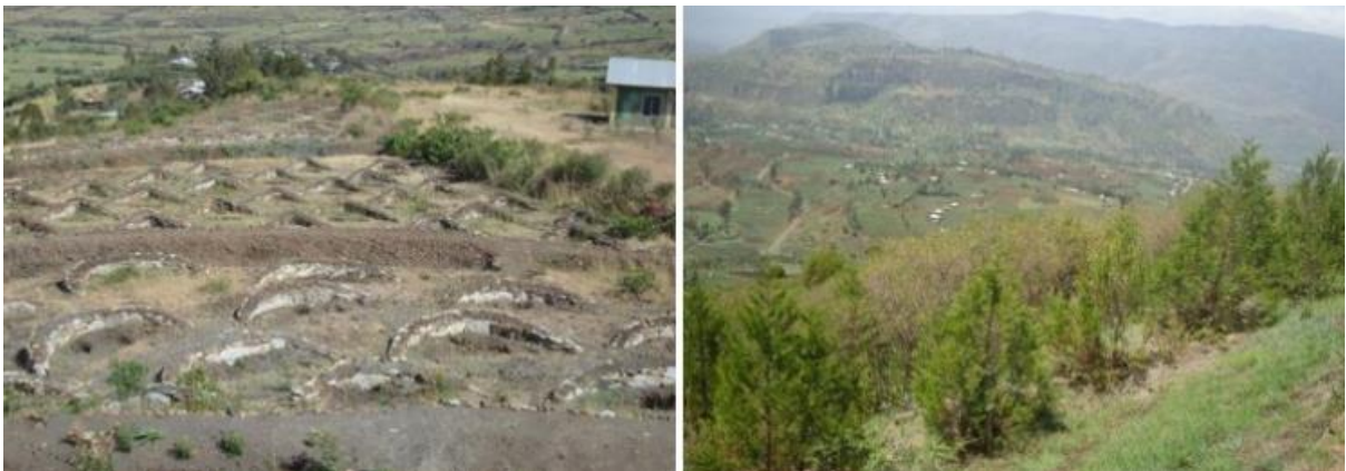
Figure 28. Eyebrow basins, trench bunds and small herring-bone basins for tree planting (same area a few years later).
