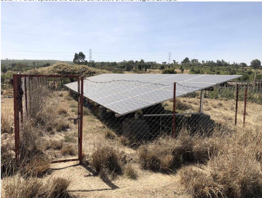
Figure 30 Solar PV that replaced the Diesel Generator, Oromia Region; Ethiopia
