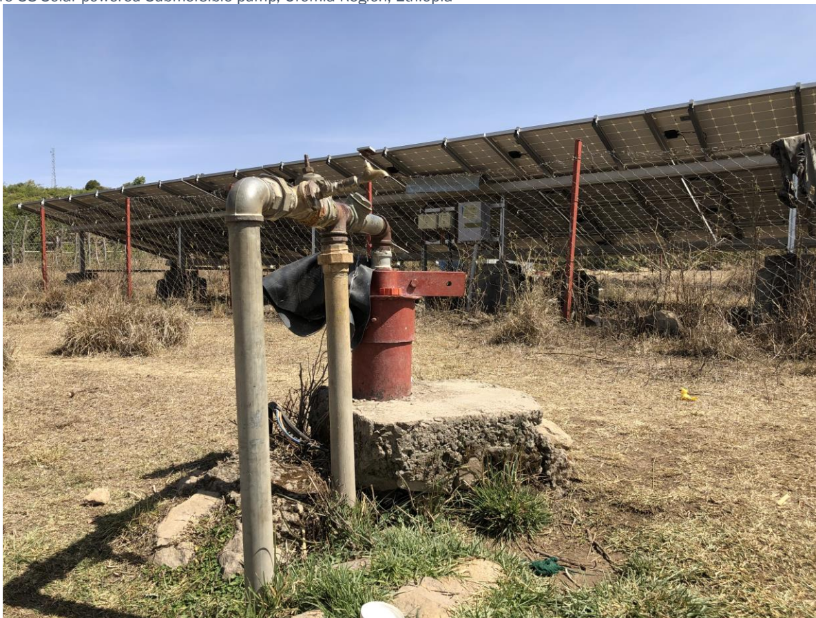
Figure 38 Solar powered Submersible pump, Oromia Region; Ethiopia
