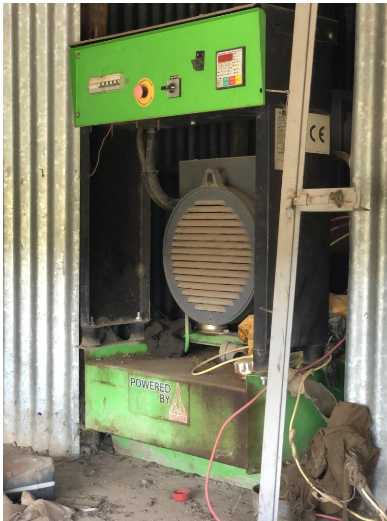
Figure 28 Diesel Generator used for borehole water extraction and replaced by Solar PV, Oromia Region; Ethiopia
