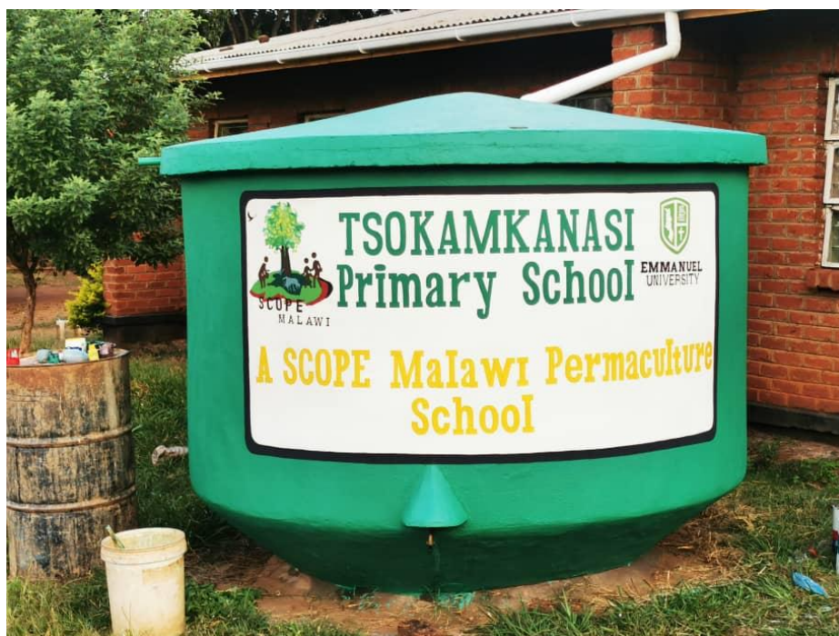
Figure 23 An example of a 10,000 litre calabash rainwater harvesting tank installed at Tsokamkanasi Primary School in Lilongwe, Malawi.
