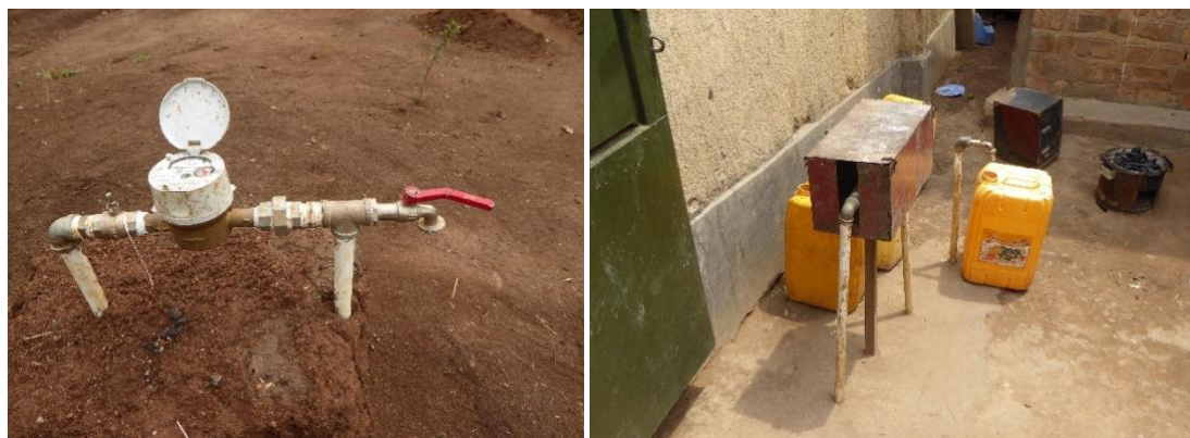
Figure 5-24: Pictures of water connections at households in the settlement. In the image on the right, the lock box is used to prevent unauthorised use of the tap.
