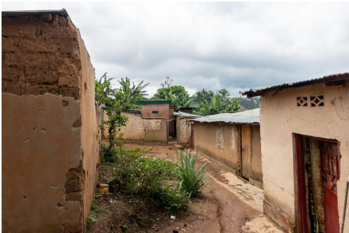
Figure 5-9: Typical part-rendered mud and clay brick facades with corrugated roofs
