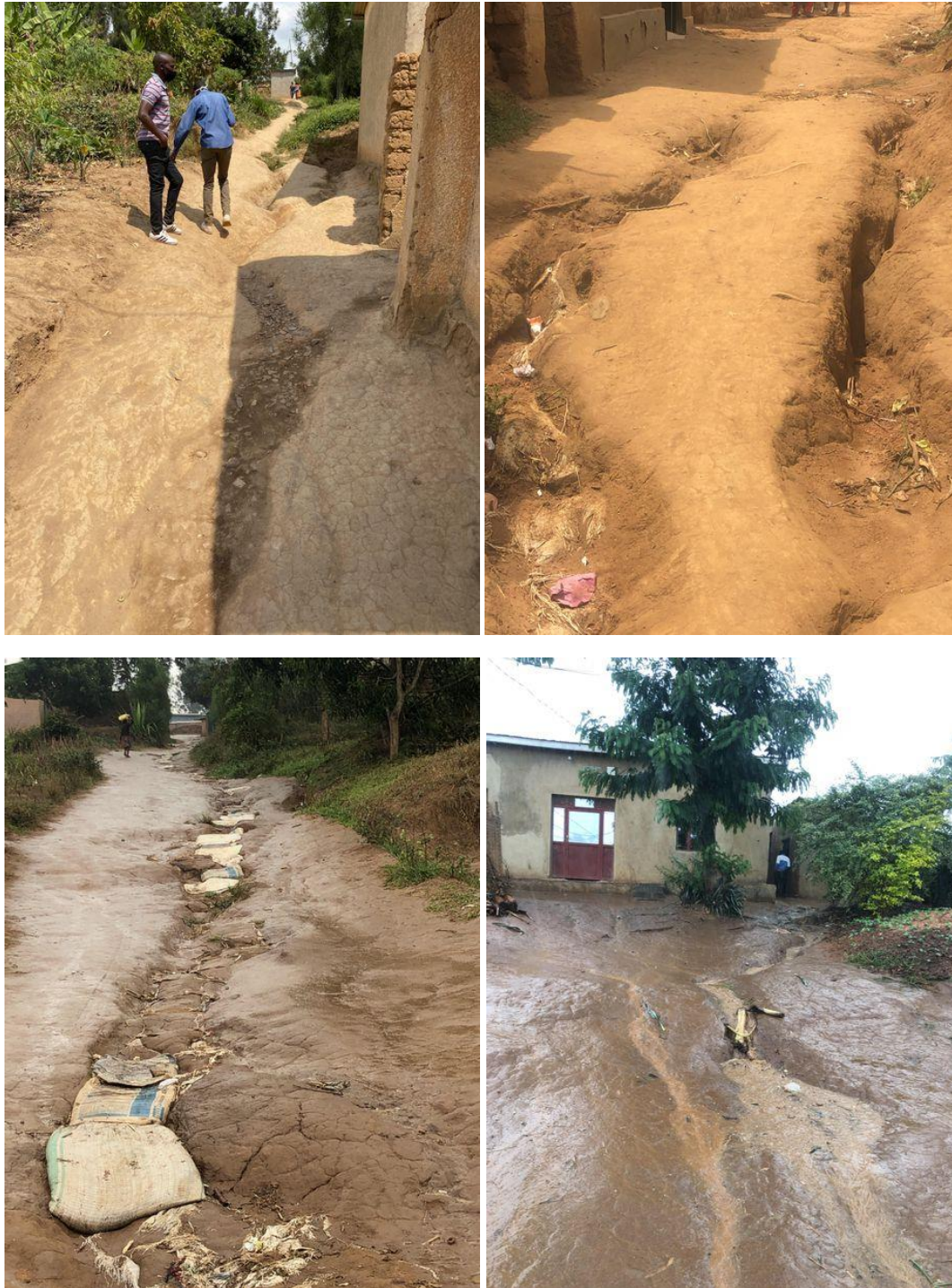
Figure 5-16: Images showing the erosion channels and slip hazards that are present throughout the settlement.
