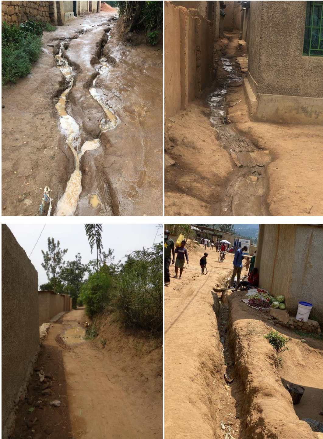
Figure 5-20: Images showing uncontrolled stormwater channels in the settlement, as well as stagnant water.
